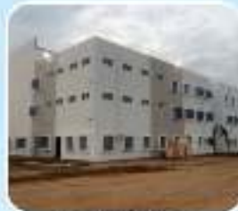
Hostel Building 26,000 Sq.ft completed in 70 days
