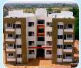
Housing for CRPF 72 Days 1 Block 251 Houses 11 Months
