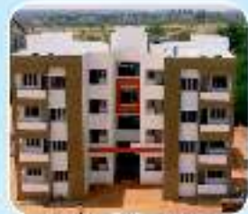
Housing for CRPF 72 Days 1 Block 251 Houses 11 Months
