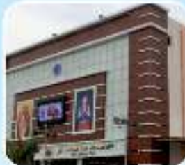
Commercial Mall 2,25,000 Sq.ft completed in 120days
