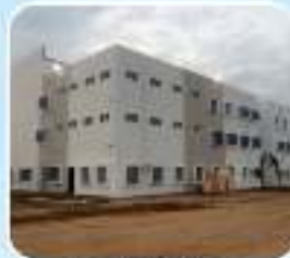
Hostel Building 26,000 Sq.ft completed in 70 days
