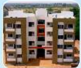
Housing for CRPF 72 Days 1 Block 251 Houses 11 Months
