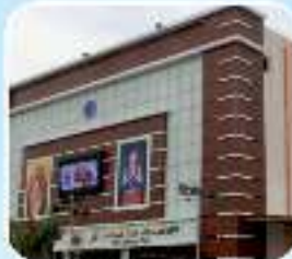
Commercial Mall 2,25,000 Sq.ft completed in 120days
