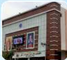
Commercial Mall 2,25,000 Sq.ft completed in 120days
