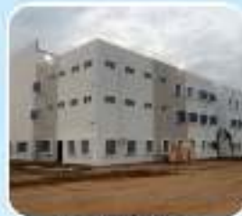
Hostel Building 26,000 Sq.ft completed in 70 days
