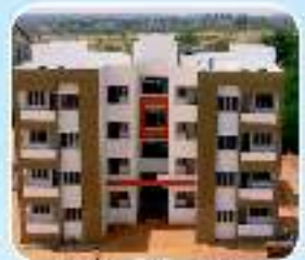
Housing for CRPF 72 Days 1 Block 251 Houses 11 Months
